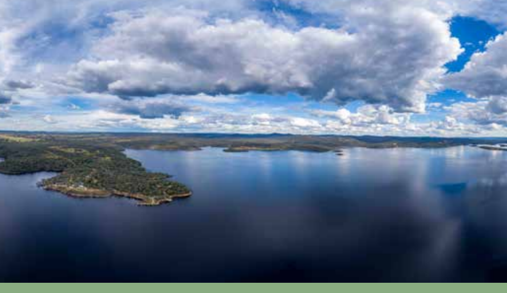
Copeton Dam, Inverell
